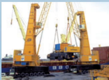
Loading pre-assembled components of a Gottwald crane
