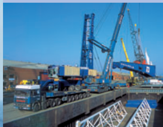
Shipping pre-assembled components of a Gottwald crane on a barge
