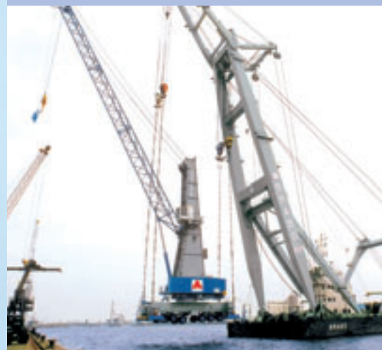
Re-locating a Gottwald crane within a port by floating crane
